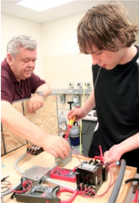
JAMIE PESOTINE/Staff Photographer James Keil, right, works with his instructor Robert Letcher testing lines as part of the Commercial Industrial Maintenance Technology course at McCann School of Business and Technology in Hazleton.
